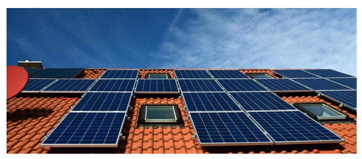
The energy produced from the photovoltaic system first satisfies the current consumption, the excess production if greater than the consumption goes to the energy storage until it is fully charged and can be used when the production stops or is lower than the demand. It is worth adding that the stored energy is available all the time. When the storage is discharged, electricity is drawn from the grid. Surplus energy can be sent to the grid.
